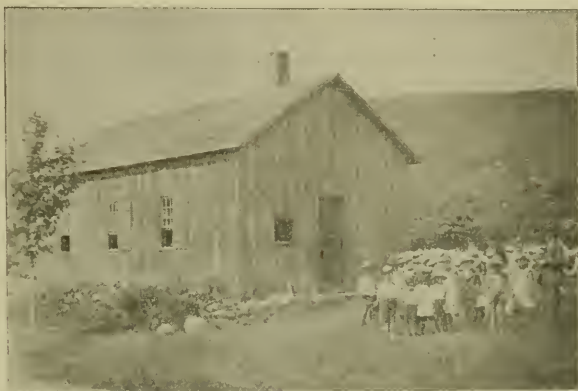
BULLS BRIDGE SCHOOL HOUSE.
